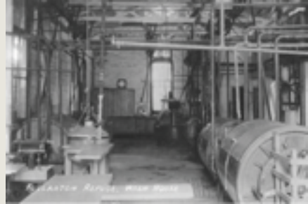
Fullarton Refuge Infirmary and Fullarton Refuge Wash House undated, Courtesy Adelaide Catholic Archdiocesan Archives.
