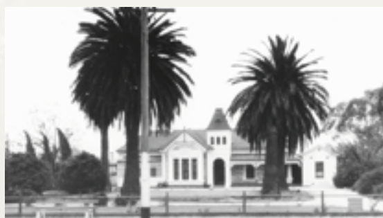
Buildings at Colebrook Quorn 1930 SLSA: B49352, Premises of the Colebrook Home for Aboriginal Children 1930 SLSA: B49356
